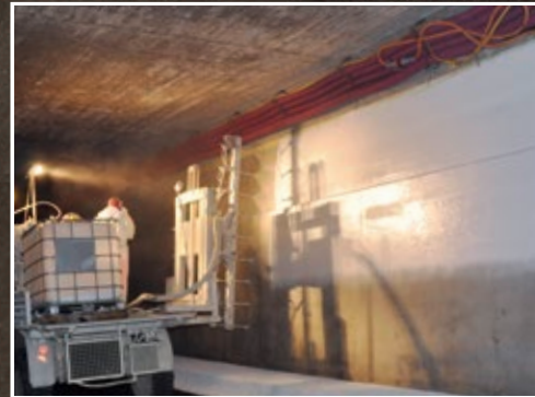
Concrete replacement and surface protection
